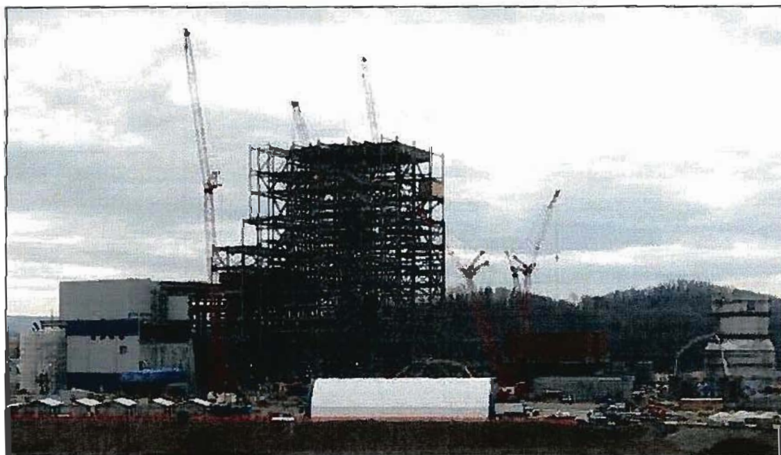
Figure 3. Boiler Structure and Flue Gas Absorber (January 2009)
