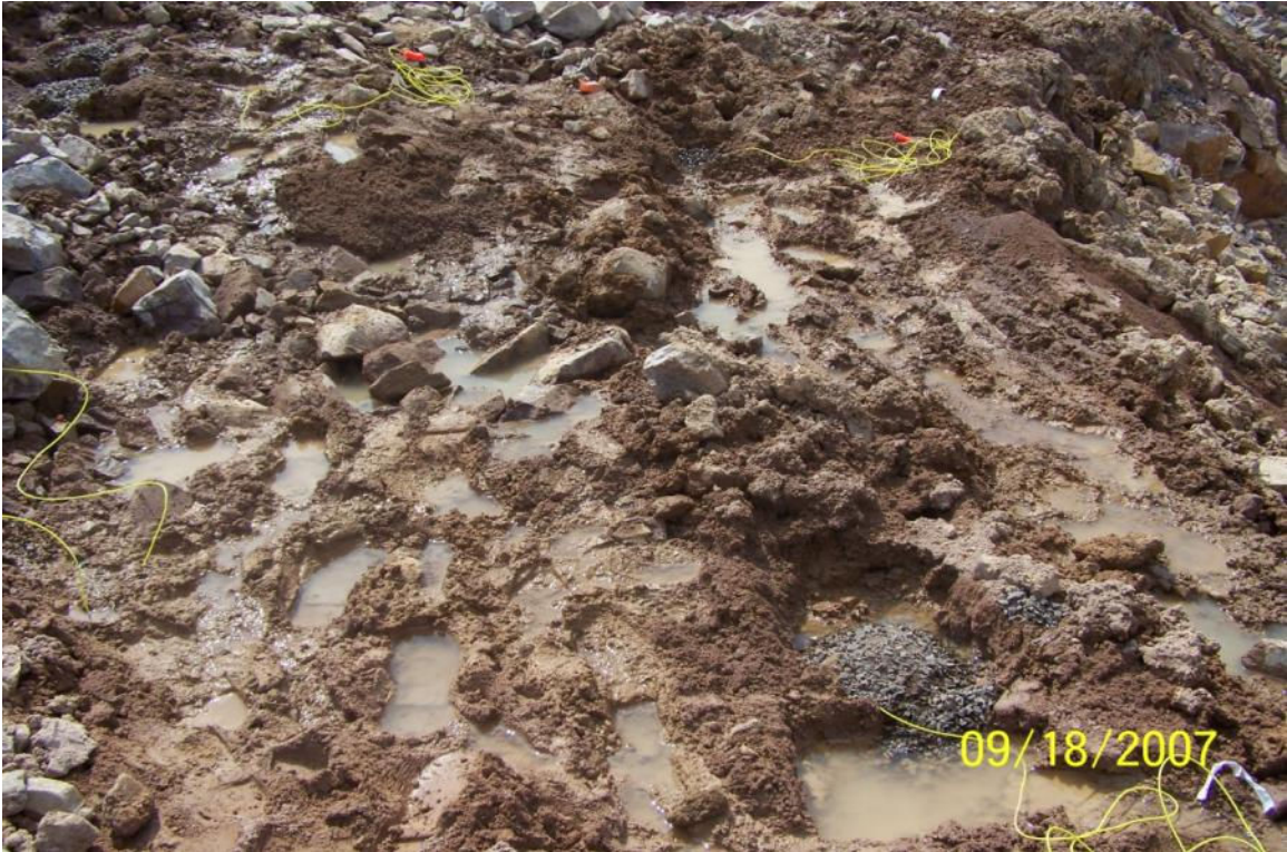
2 SILTY CLAYEY SAND AT THE ORIGINAL FOUNDATION ROCK INTERFACE
