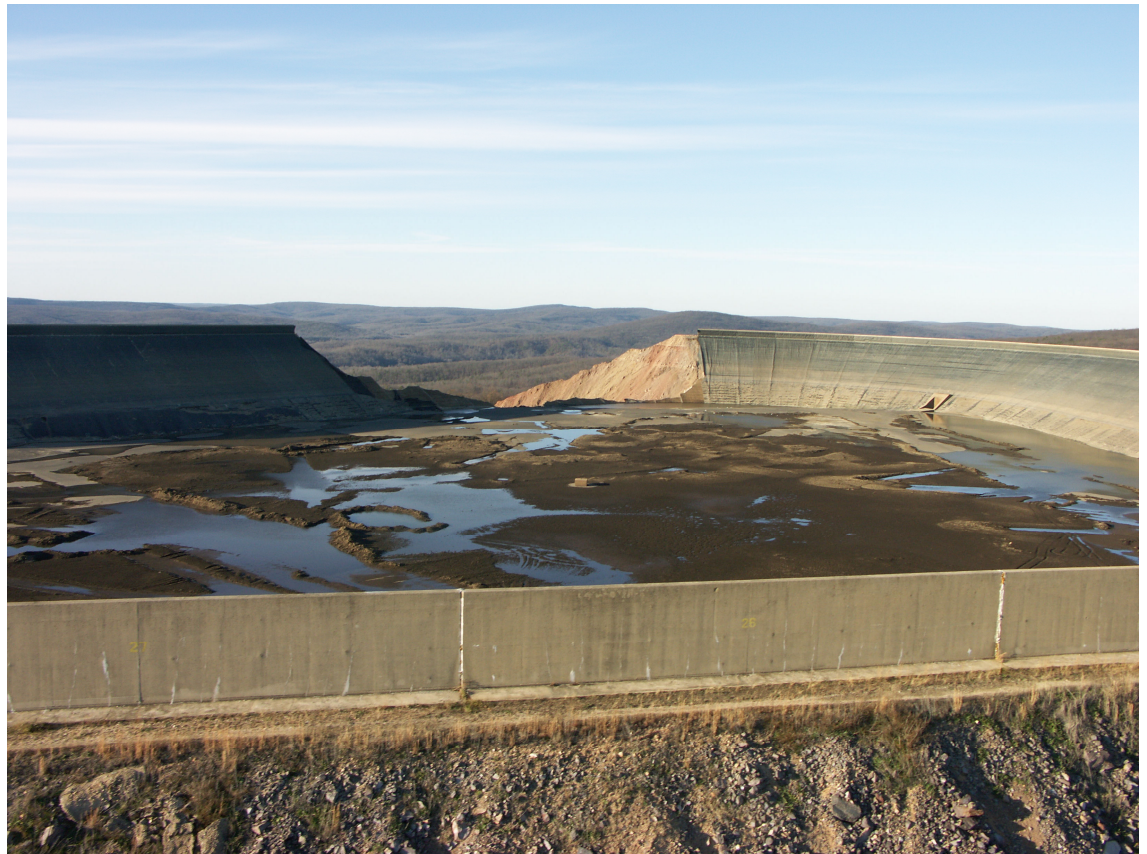
OLD PARAPET WALL AS IT APPEARED AFTER THE BREACH
