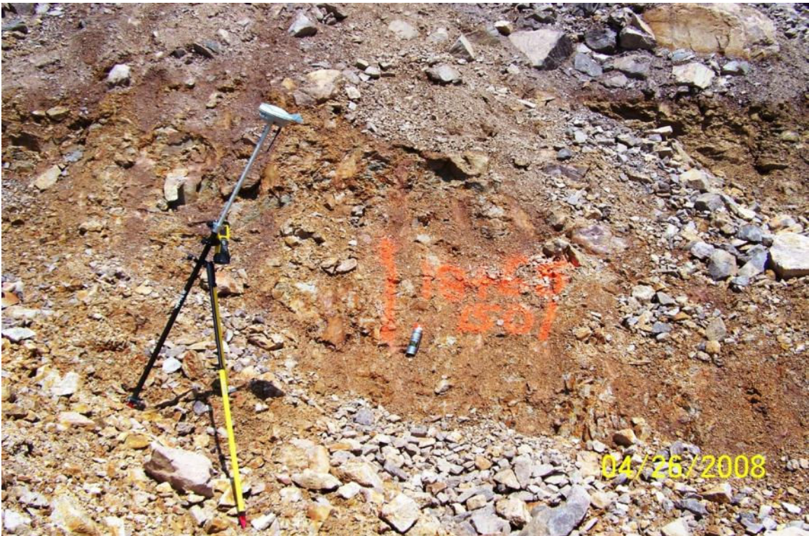
4 CLAYEY MATERIAL AT ORIGINAL FOUNDATION ROCK INTERFACE
