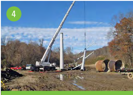
4 Lift and place structure on foundation
