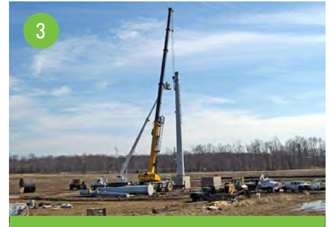
3 Assemble structure on the ground
