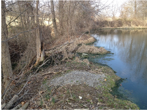
Old Lagoon Untreated Waste Draining into creek
