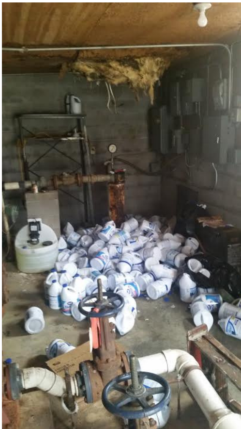
Original Brandco Well House
