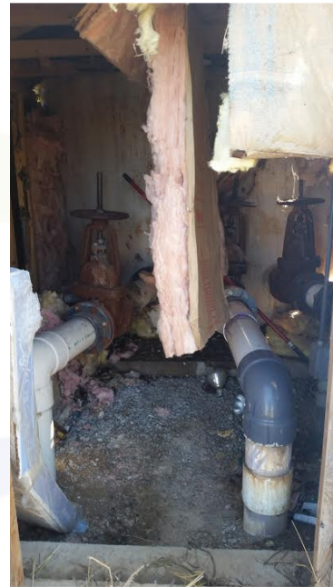
Looking Down Roof Hole over Drinking Water Well Head
