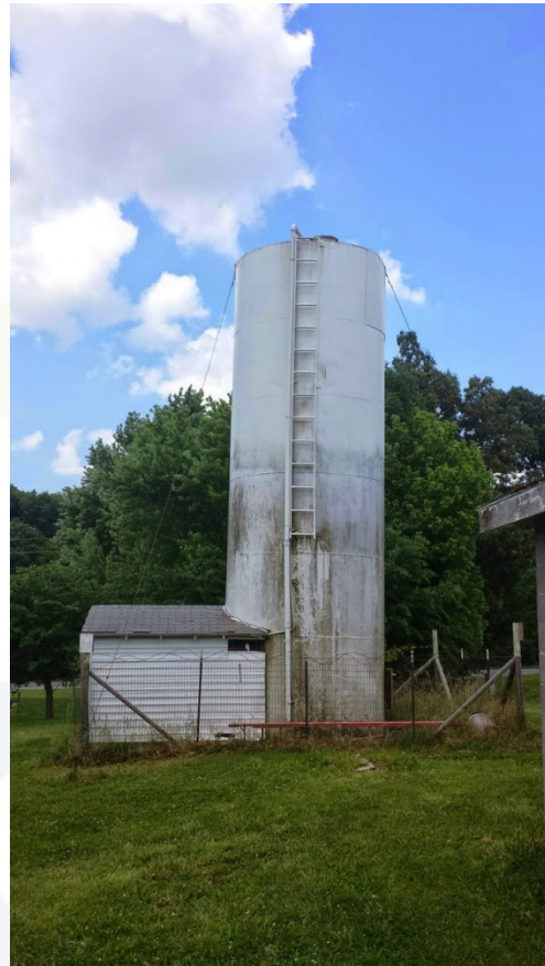
Original Brandco Tower
