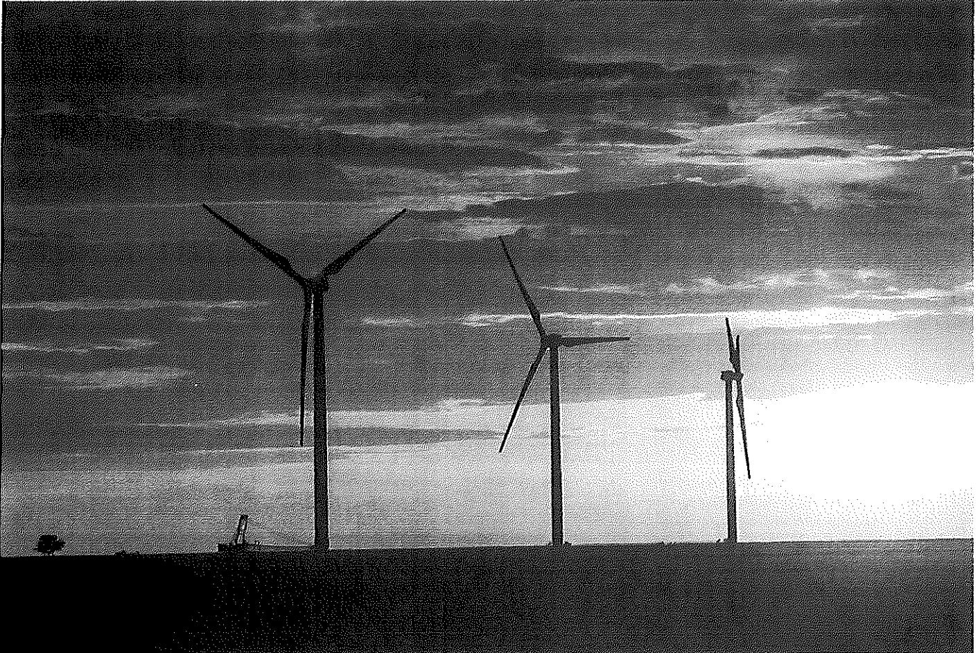
Energy's Flat Ridge Wind Farm in Kansas (photo submitted).
