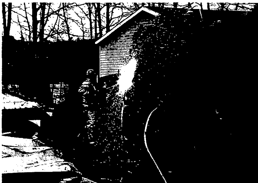
3. Oxy-lance cutting of individual components—such as these pump house water boxes—expedite site cleanup
