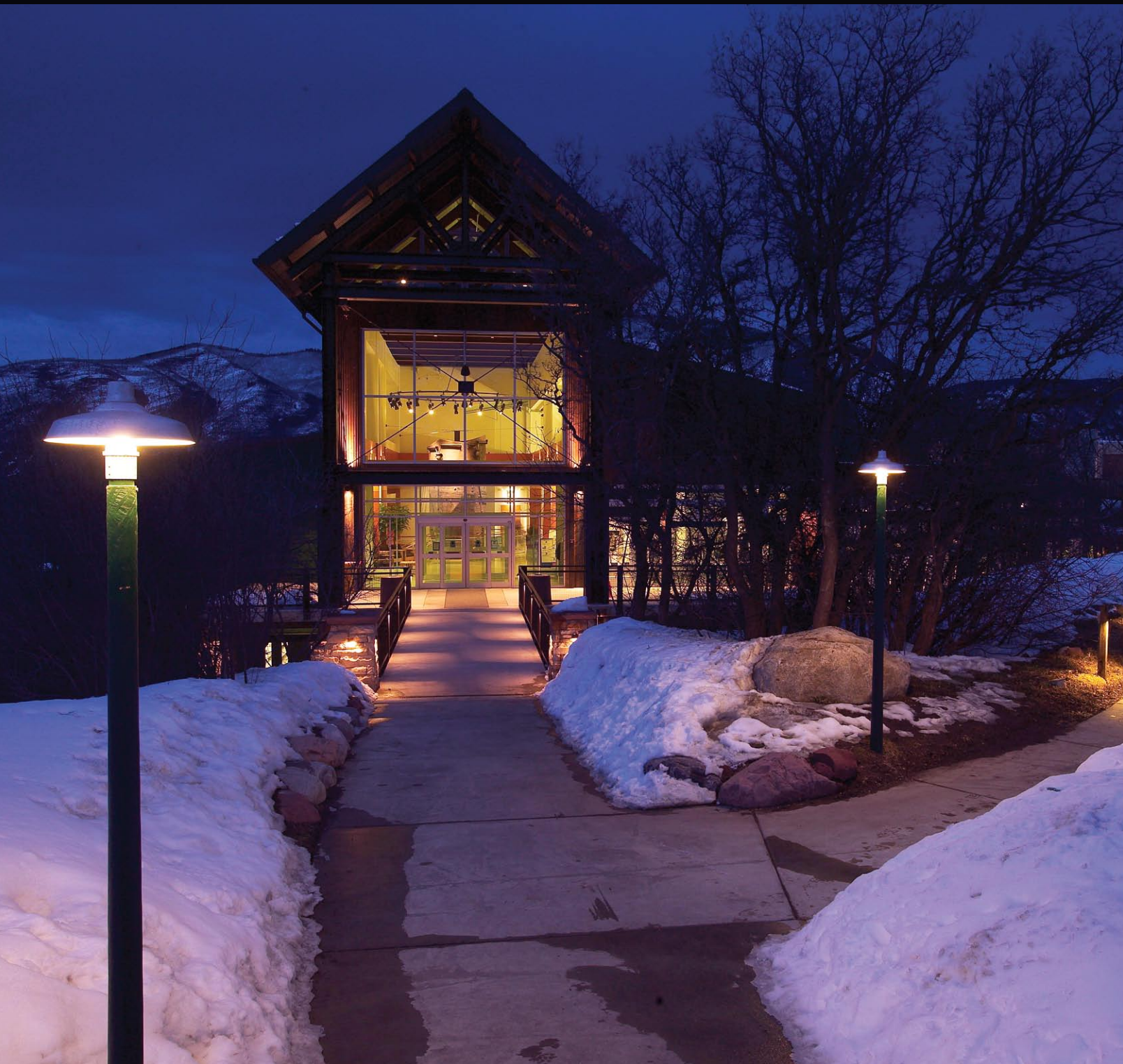
The Aspen Recreation Center in Aspen, Colorado, won the 2004 IDA Lighting Design Award. The award recognizes lighting designs that are free of glare, use optimal levels of light, are energy-efficient, and provide pleasant ambience with minimal obtrusive light and contribution to sky glow. Lights that are fully shielded and well spaced keep light where it is directed, minimizing light pollution.
