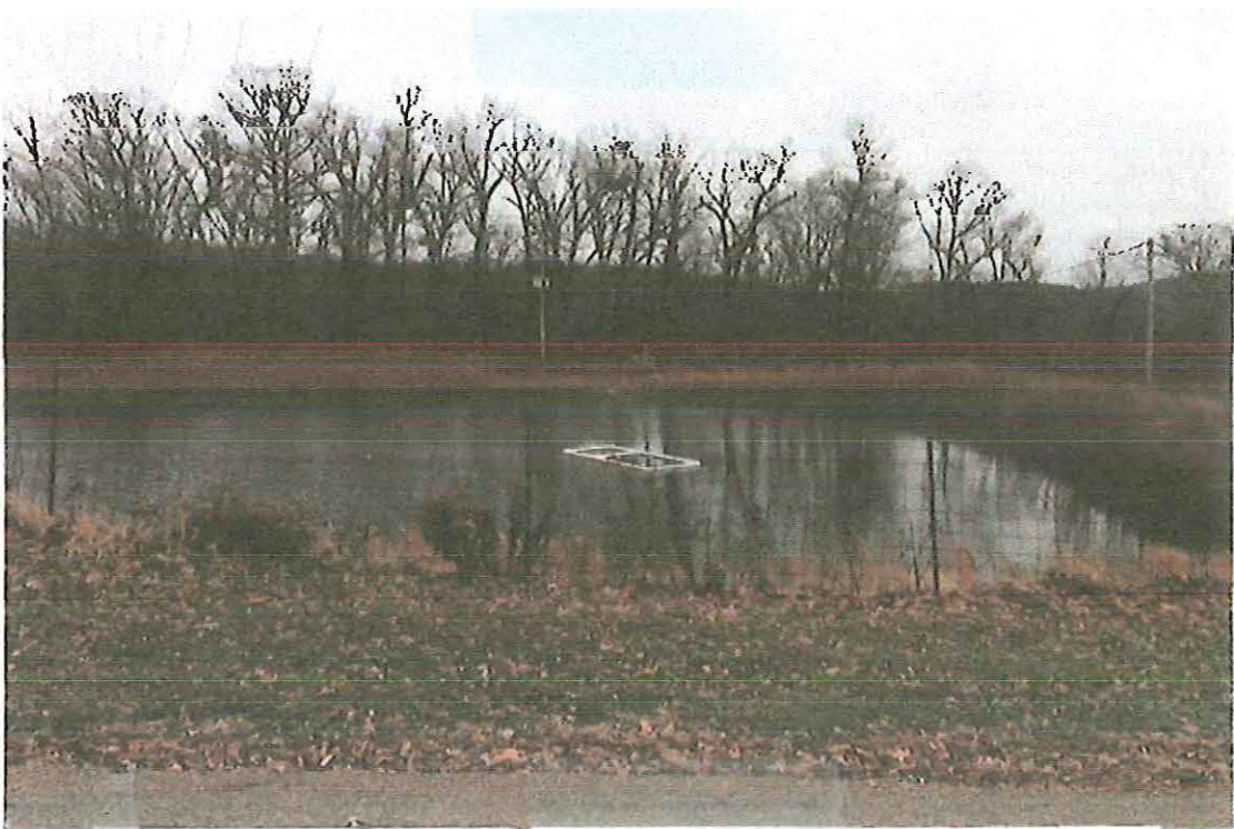
Cell 4 of Lagoon and Irrigation Intake
