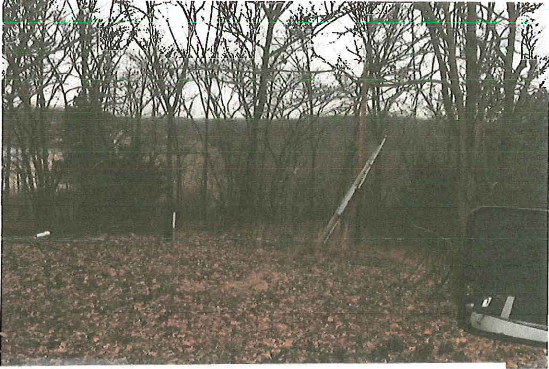
Well #2 open Well Head
