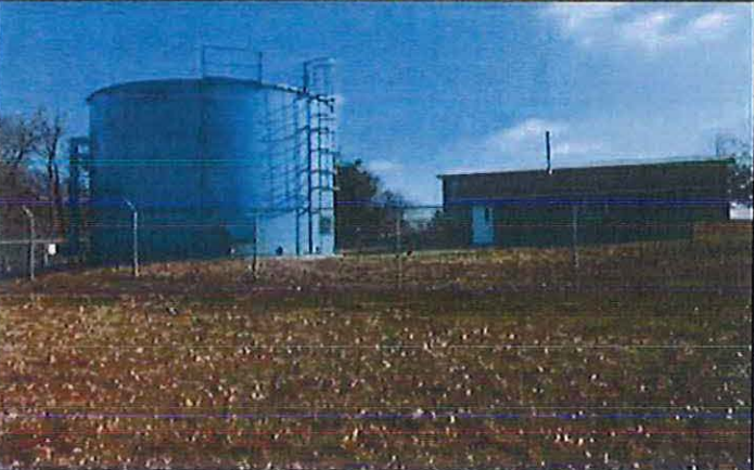
Photo #: 008 Date Taken: 01/24/2018 By: Michael Wyatt Program: PDWB File: Hillcrest Utility Operating Co., Inc. – General Location: Well/tank site Description: Fenced well house and storage tank.
