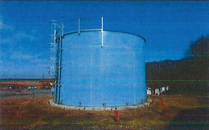
Photo #: 007 Date Taken: 01/24/2018 By: Michael Wyatt Program: PDWB File: Hillcrest Utility Operating Co., Inc. – General Location: Tank site Description: 58,000 gallon ground storage tank.
