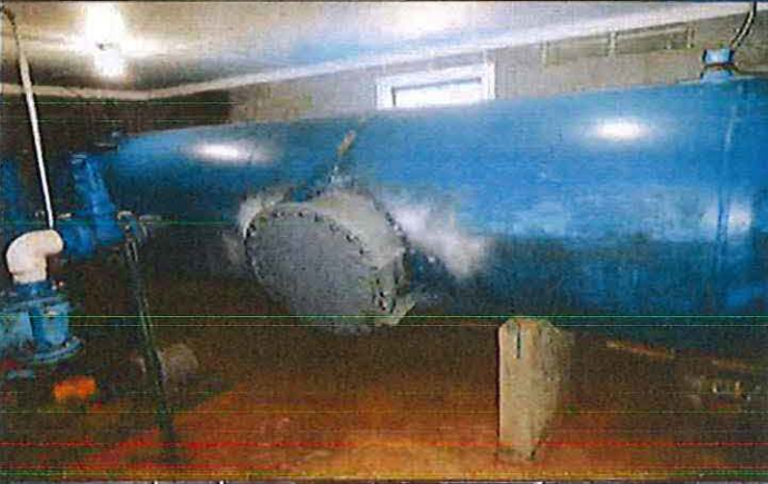
Photo #: 003 Date Taken: 01/24/2018 By: Michael Wyatt Program: PDWB File: Hillcrest Utility Operating Co., Inc. – General Location: Well house Description: ~2,100 gallon hydro-pneumatic pressure tank.
