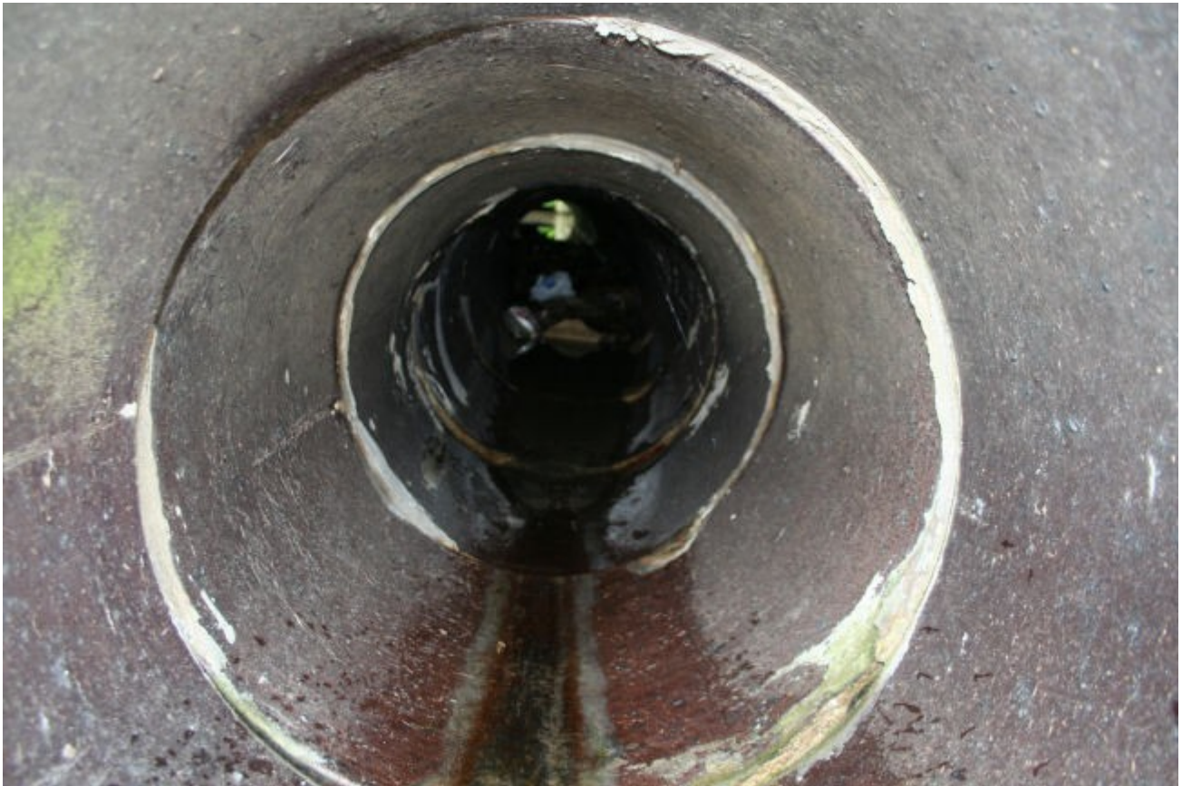
Above three pictures. Water still flowing into the 2 foot drain tile at Larimore and McQuay.
