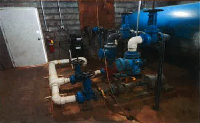
Photo #: 004 Date Taken: 01/24/2018 By: Michael Wyatt Program: PDWB File: Hillcrest Utility Operating Co., Inc. – General Location: Well house Description: High service pumps.
