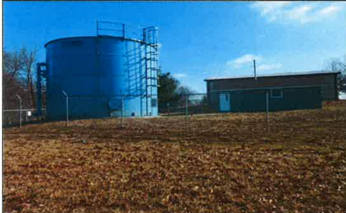
Photo #: 008 Date Taken: 01/24/2018 By: Michael Wyatt Program: PDWB File: Hillcrest Utility Operating Co., Inc. – General Location: Well/tank site Description: Fenced well house and storage tank.
