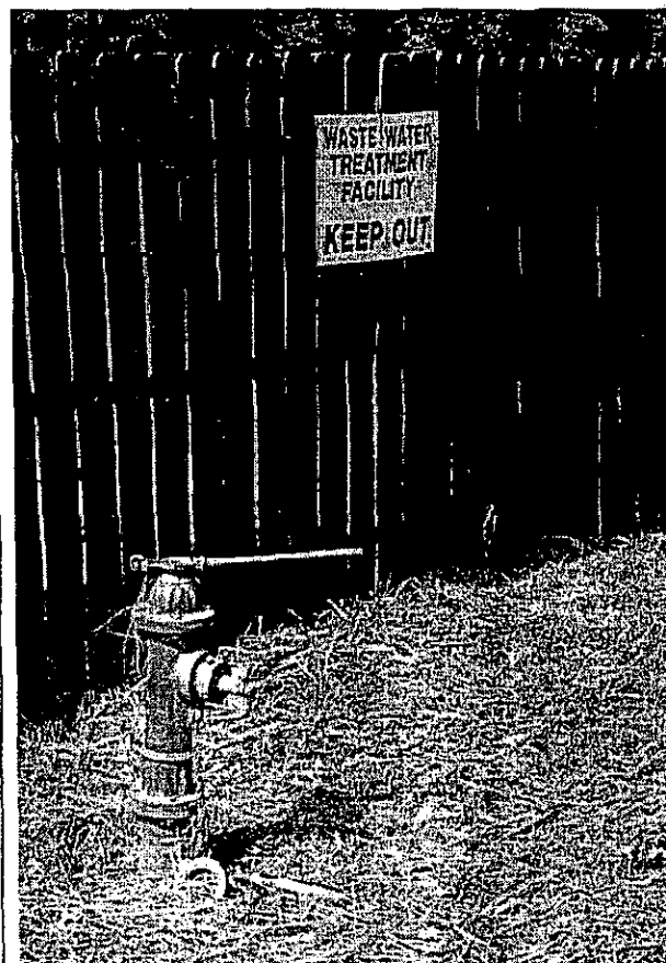
Figure 3: Hose connected to hydrant used inside wastewater treatment plant. No backflow prevention assembly in use.
