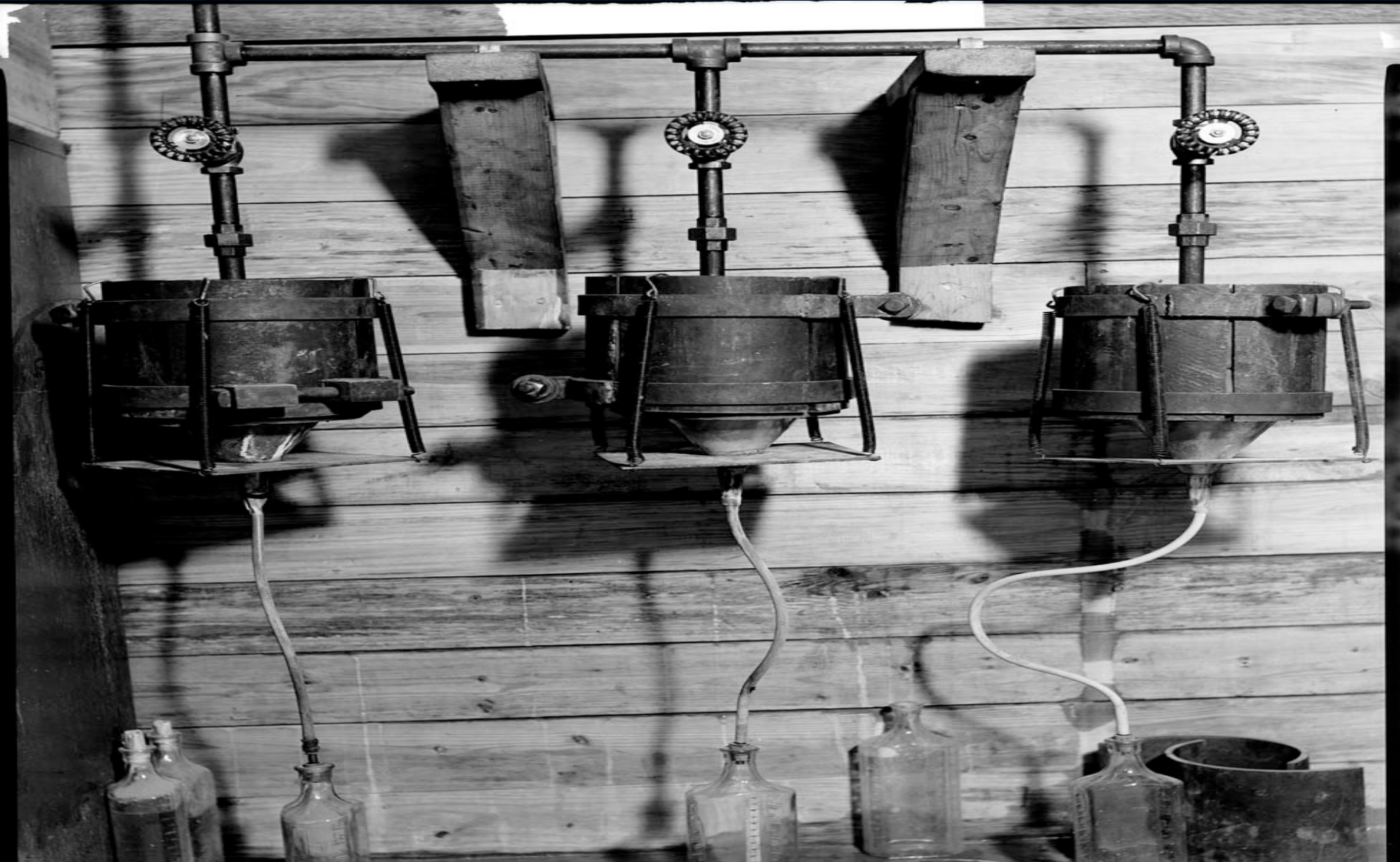
UNION ELECTRIC LIGHT & POWER Co. - HYDROELECTRIC STATION - OSAGE DEVELOPMENT STONE & WEBSTER ENGINEERING CORPORATION, Builders J.O. 5461 * 287, 8-27-30 Concrete Laboratory, Close-Up of Apparatus for Permeability Tests of Concrete Blocks N2141
