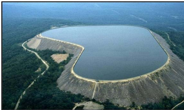
ORIGINAL UPPER RESERVOIR CONCRETE FACED ROCKFILL DAM
