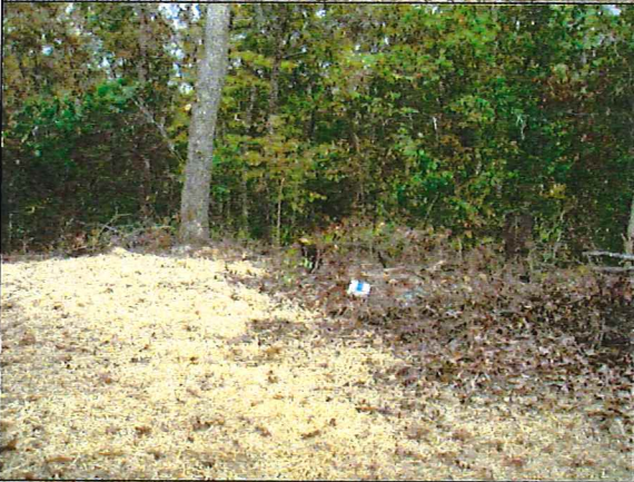
Photo #:010 Date Taken: 10/26/2016 By: Michelle Oglesby Program: PDWB File: Crawford County Location: Indian Hills Utilities Operating Co. Inc. Description: Location where Well #2 booster pumps station was located.
