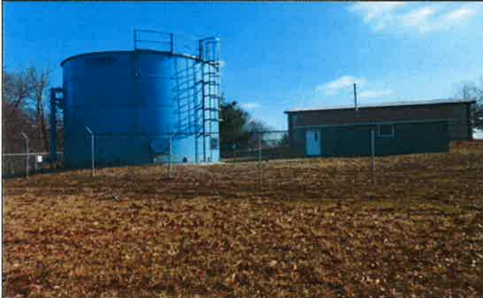
Photo #: 008 Date Taken: 01/24/2018 By: Michael Wyatt Program: PDWB File: Hillcrest Utility Operating Co., Inc. – General Location: Well/tank site Description: Fenced well house and storage tank.
