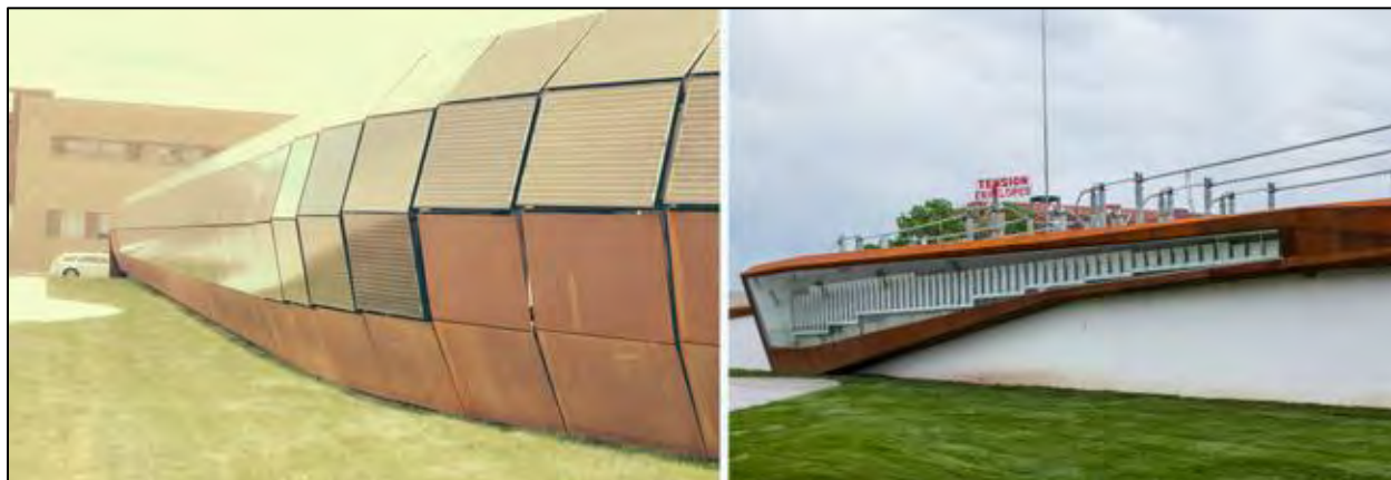
Figure 3-138: Crosstown Substation Solar Installation
