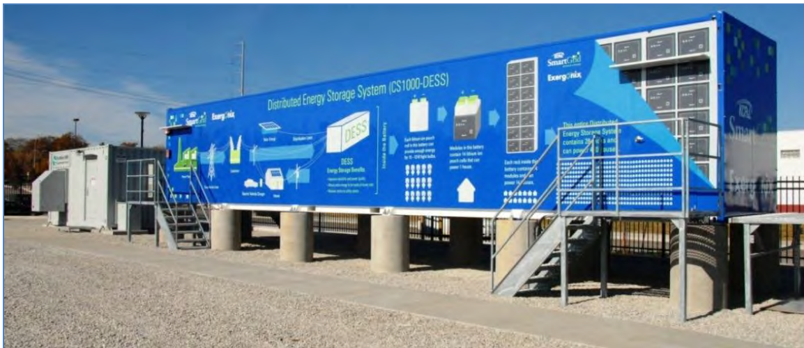
Figure 1-27: Grid-Connected Battery
