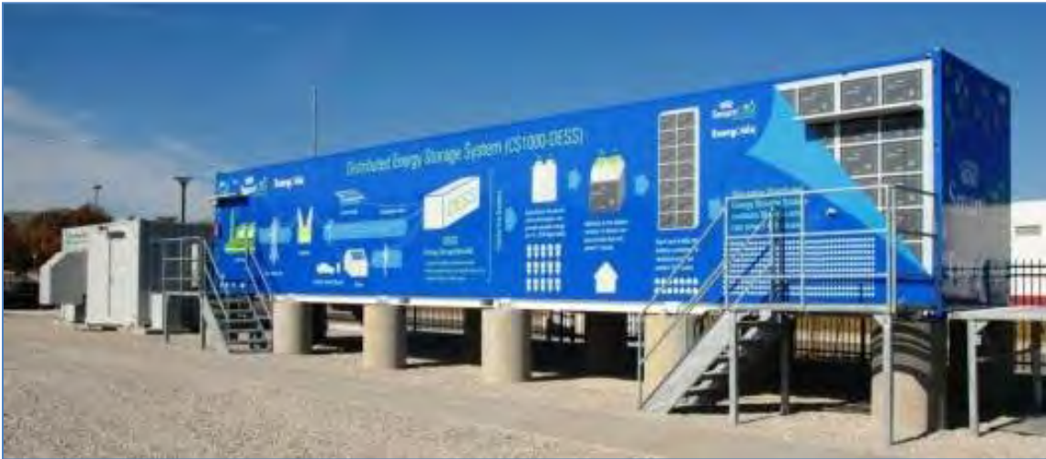
Figure 2-73: BESS Installation
