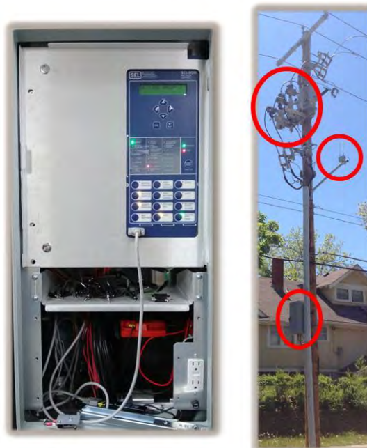
Figure 2-65: Typical Recloser Installation
