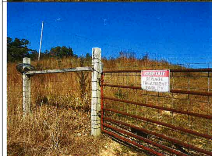
Photograph #: 011 Taken by: Elizabeth Stephens Entity: Confluence Rivers-Port Perry WWTF Permit: MOG823126 Location: Perry County Description: View of one gate from the fenced enclosure. Note sign on gate. Date Taken: October 1, 2020 Program: WPC Unit
