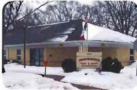
Independence Light & Power, Telecommunications office facility.
