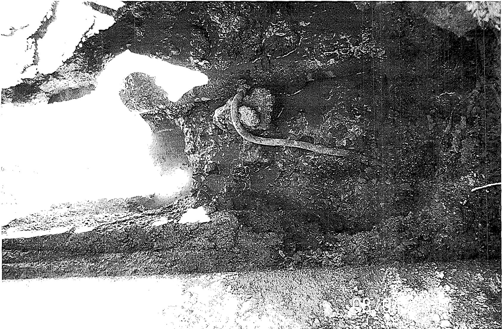
Pictured here is a lead service line connected to an old four-inch cast iron water main, appearing near the top of the picture. The old main is being replaced with a new eight-inch PVC water main, appearing at the bottom of the picture, and the lead pipe portion of the service line will be replaced with new copper pipe.
