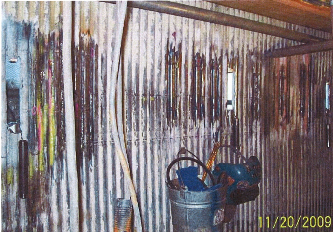
Alstom – Front Wall Welding New Tube Section
