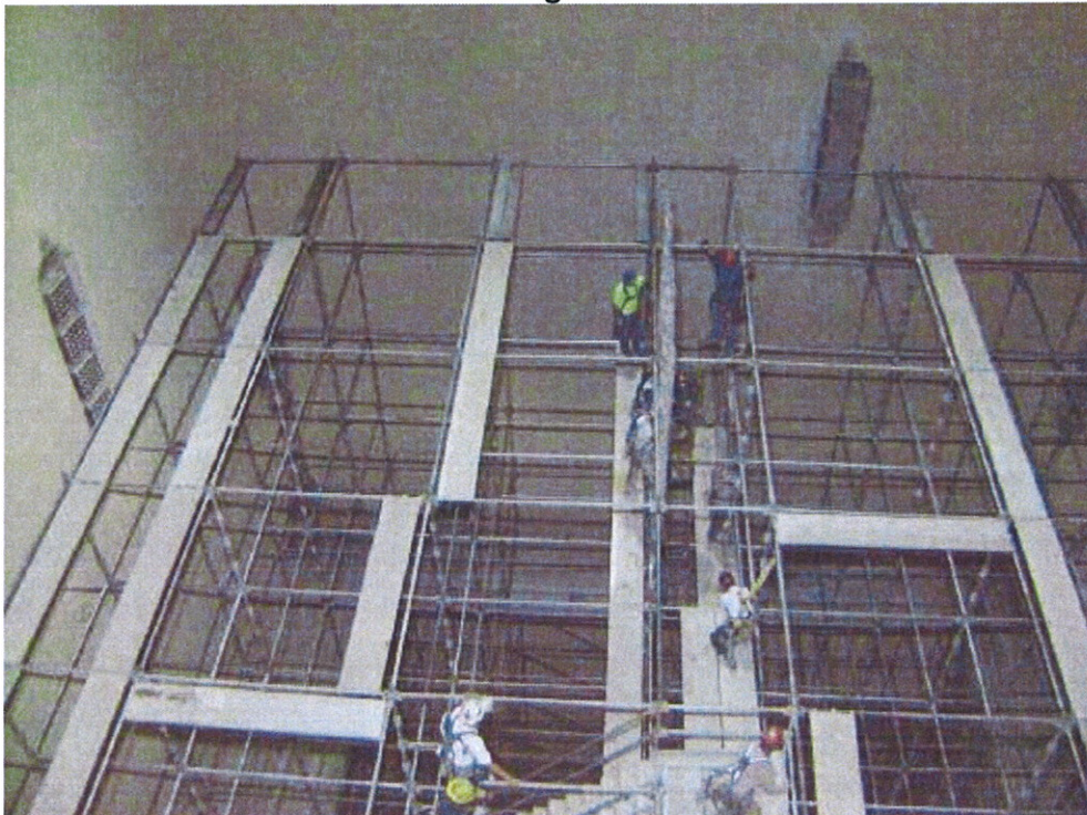
Alstom – Scaffolding Inside the Furnace
