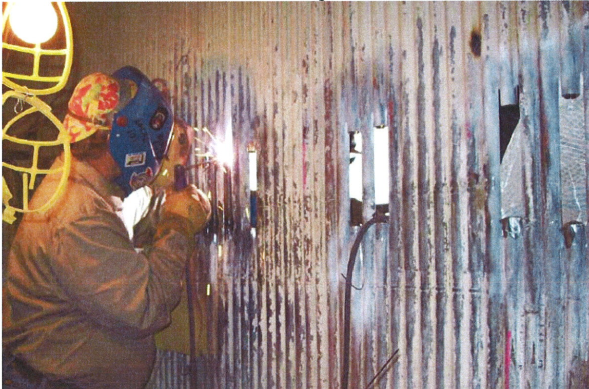
Alstom – Front Wall Welding New Tube Section
