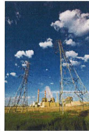
Expand Image Comanche transmission towers.
