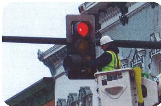
Routine maintenance on traffic lights.
