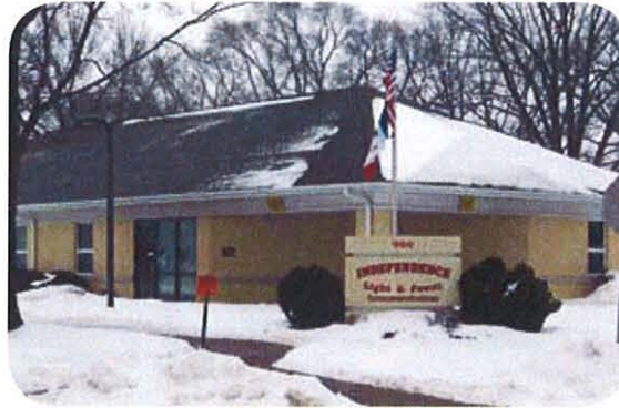
Independence Light & Power, Telecommunications office facility.
