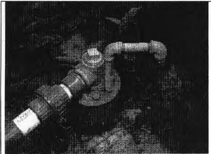
Location: Taney Co Water LLC – Venice Photographer: Katie Hirtz Photograph Date: December 10, 2014 Comments: Valley View well. Caulk needs to be applied between the top casing plates.
