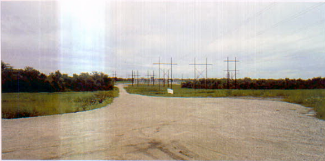
Photo No. 1 – View from the site boundary (property line) looking south from the corner of 203 rd St. and the substation access road.
