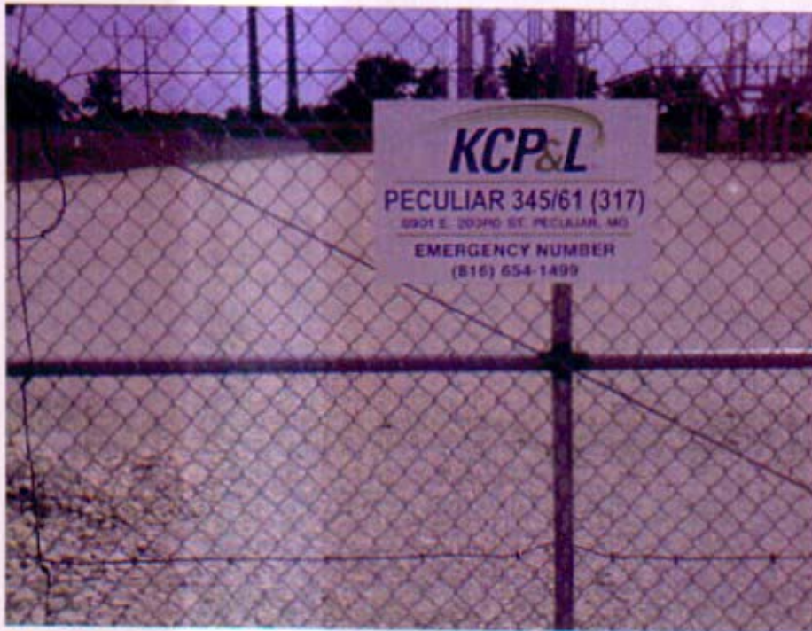
Photo No. 5-5: KCP&L Identification Sign on Substation Perimeter Fence Gate
