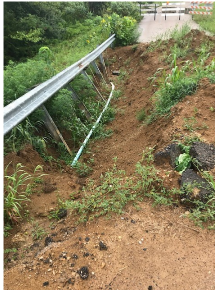
Force main exposed by road washed out from dam
