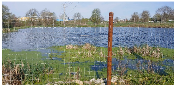
Fencing around lagoon and aeration visible in lagoon
