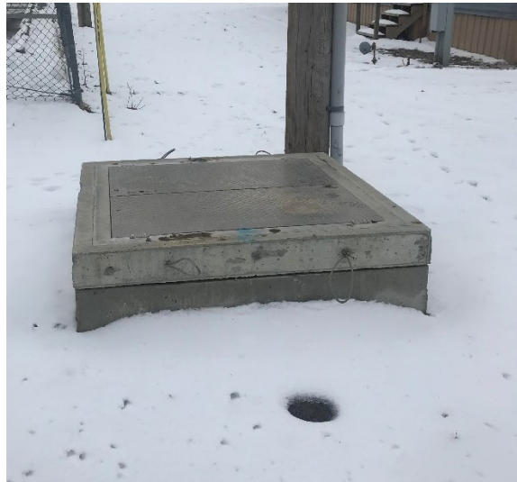
Valve vault with PRV with emergency supply from City of Sedalia
