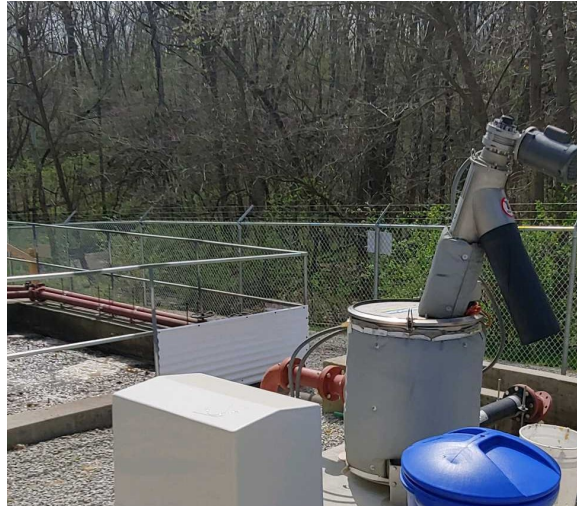
New screw screen and mixing blower
