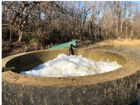
New MBBR at startup (note foaming lasted first few days)
