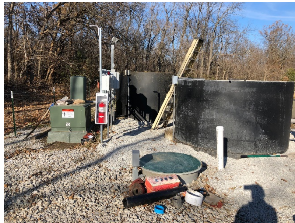
New tankage, power supply and lift station
