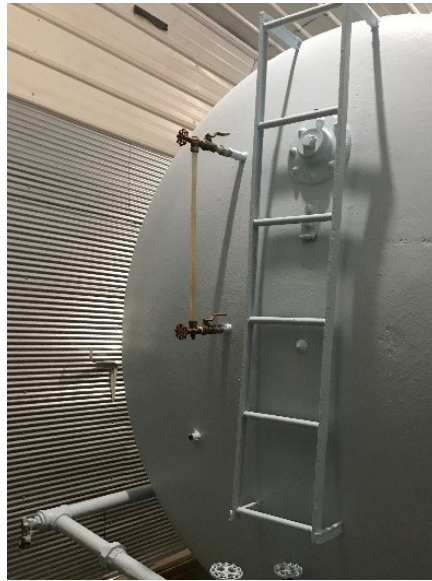
Tank exterior recoated and new tank monitoring equipment installed
