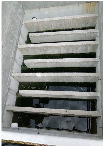
New chlorine contact chamber
