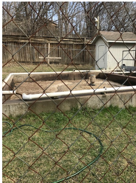
Aeration basin with single surface aerator, also PVC piping visible
