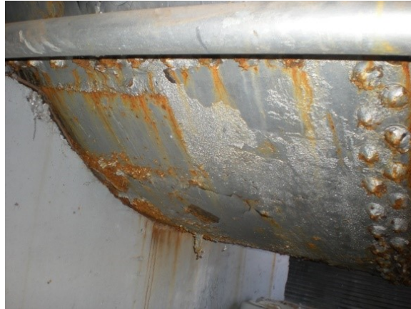
Leaking and rust on hydropneumatic storage tank exterior
