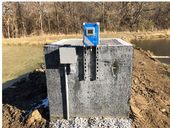
New weir box and flow meter
