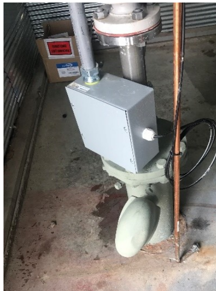
Reworked well head and new monitoring equipment
