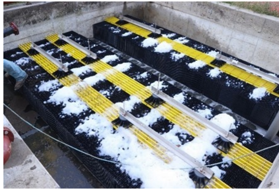
IFAS media visible during construction
