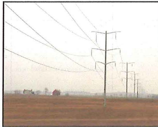
Figure 2 Typical Single-Pole, Double-Circuit Structure
