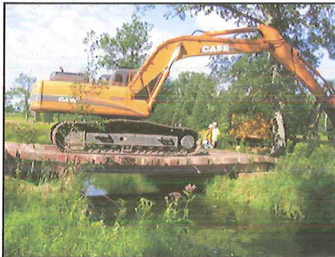
Figure 5 Temporary Bridge Structure Spanning a Waterway
