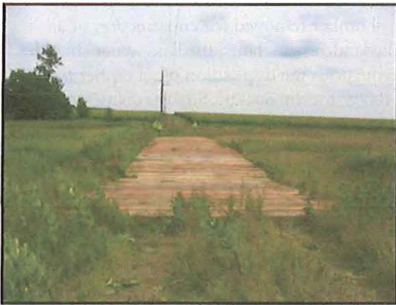
Figure 7 Mats Used in a Wet Meadow
