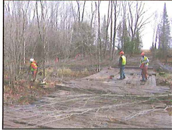
Figure 10 Hand Clearing Channel
