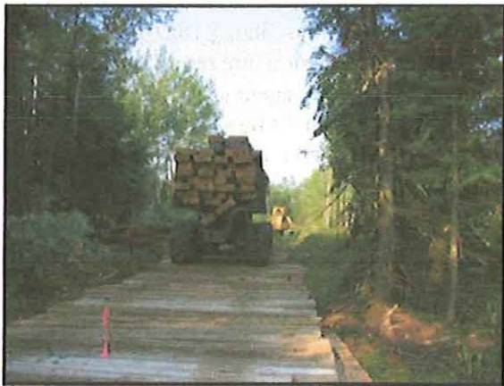
Figure 8 Mats Used in a Wooded Wetland
