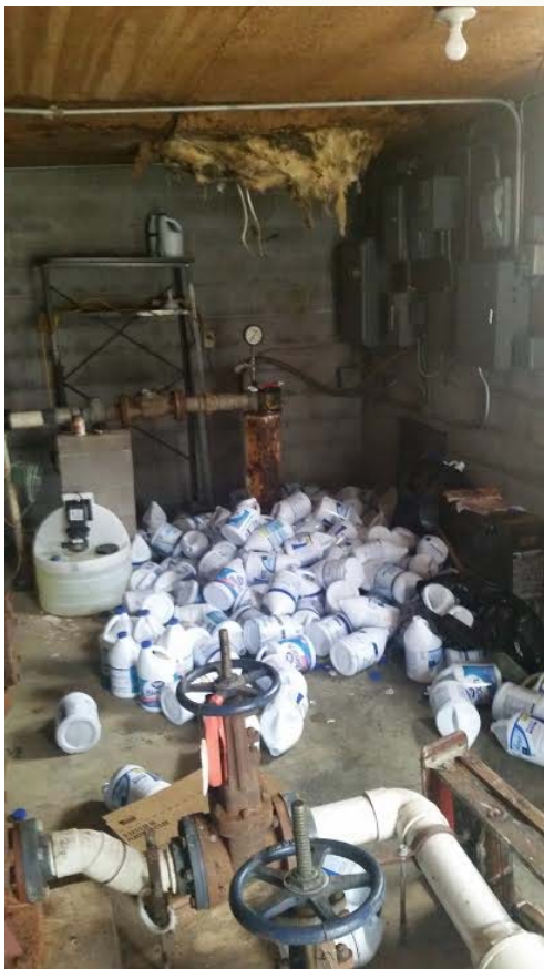
Original Brandco Well House
