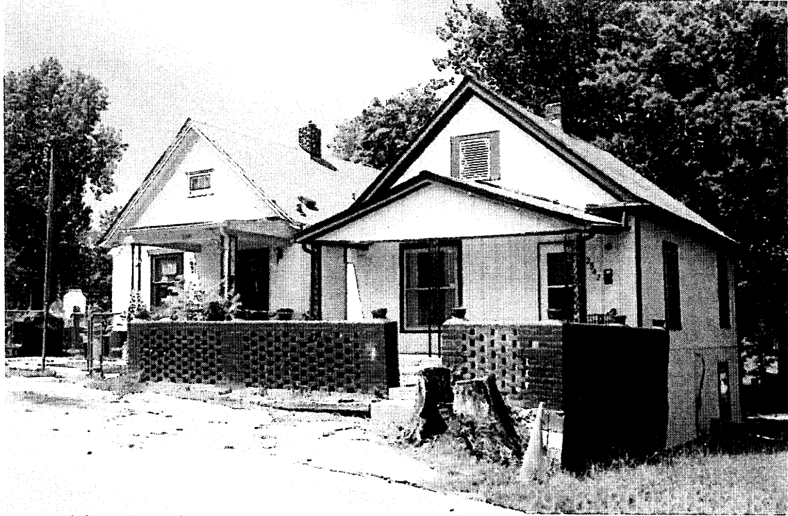
Tracts 6 (left) and 7 (right). Note possible asbestos containing exterior siding material on Tract 7 (2544 Bellevue).
