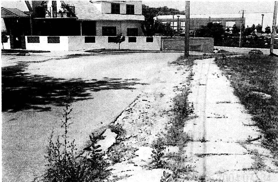
Deteriorated sidewalk and curb system along southern boundary of the Planning Area. Tract 9 to the right.
