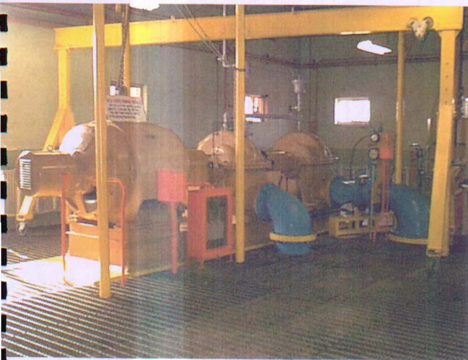
PUMP WITH HOIST AVAILABLE
