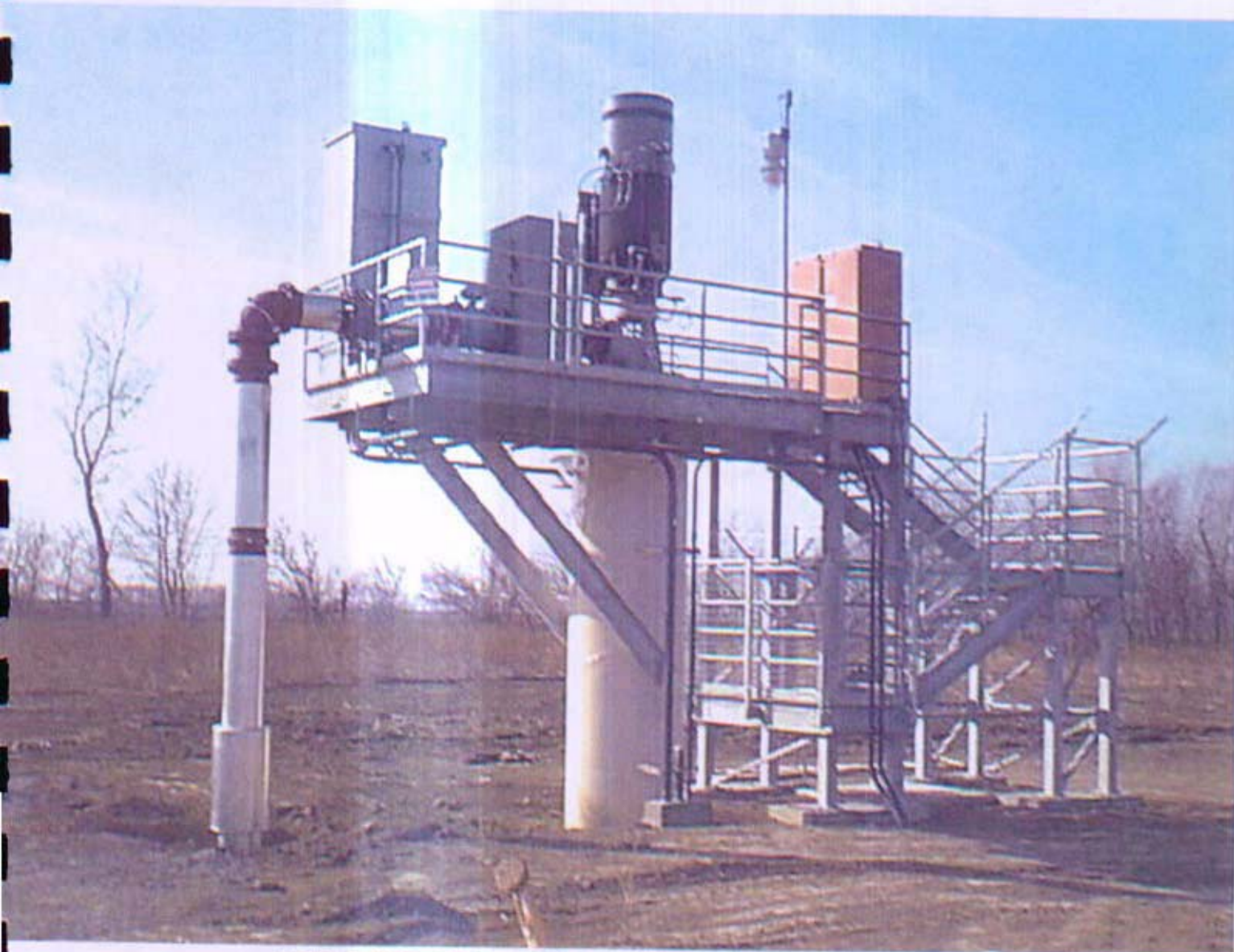
NEW 3 MGD WELL, ONE OF SEVEN, ALL IDENTICAL
