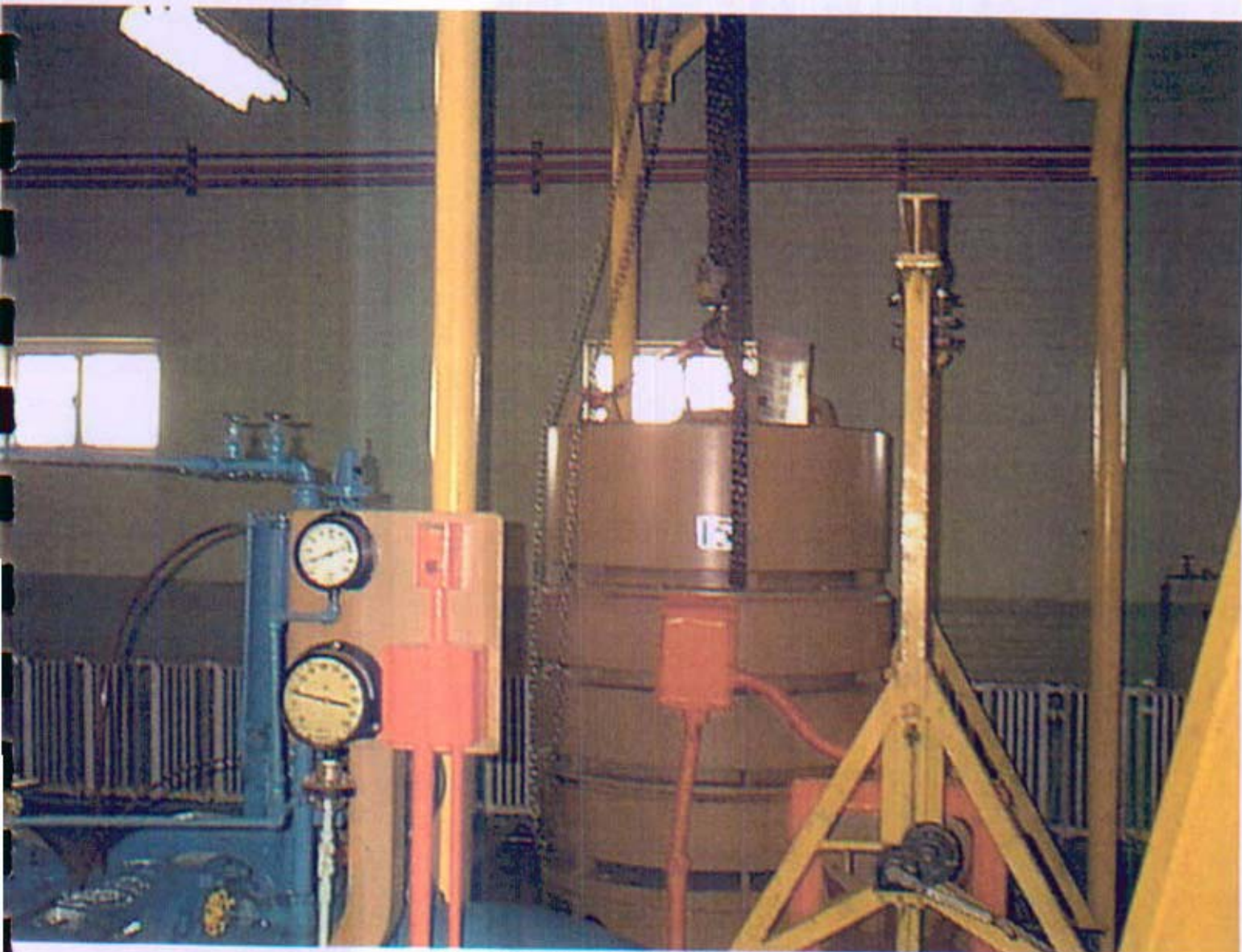
PUMP WITH HOIST AVAILABLE
