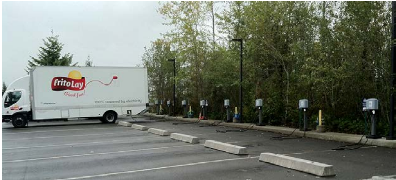
Photo 19. Fleet EVSE at Frito Lay Depot in Federal Way, Wash. Photo from Mike Simpson/NREL, NREL 29587.
