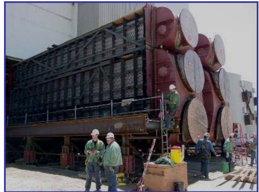
New Condenser Tube Bundle
