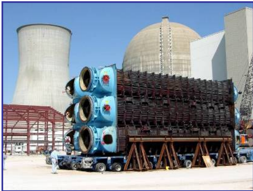
Old Condenser Tube Bundle
