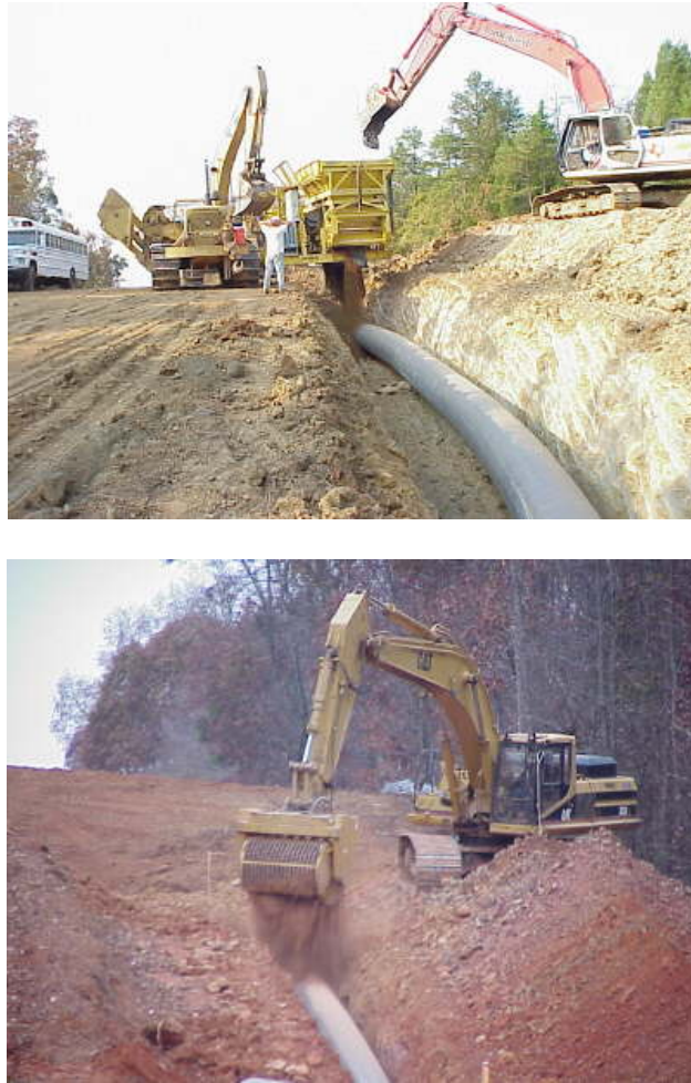
FIGURE 3.3-14 Backfilling Pipeline (Source: Photos courtesy of U.S. Pipeline, Inc. Reproduced with permission.)
