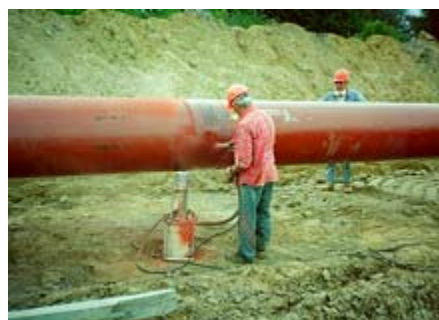
FIGURE 3.3-12 Applying Coating to Pipeline
