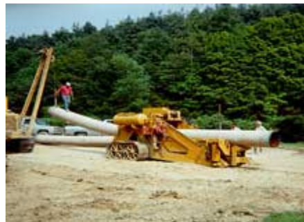
FIGURE 3.3-11 Pipe Bending Machine
