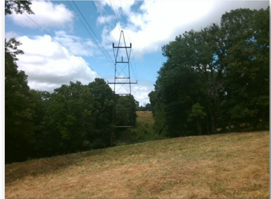
Figure 1: A-Frame Structure Configuration used on Line 69-0
