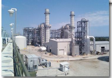
The basic Dogwood power generating process combines two combustion turbine engines and a boiler/steam turbine into a "combined cycle" that generates electricity about 30% more efficiently than conventional coal-or oil-fired plants with far less environmental impact.
