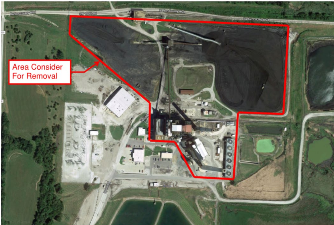
4 5 Figure 1 – Facilities Identified for Demolition
