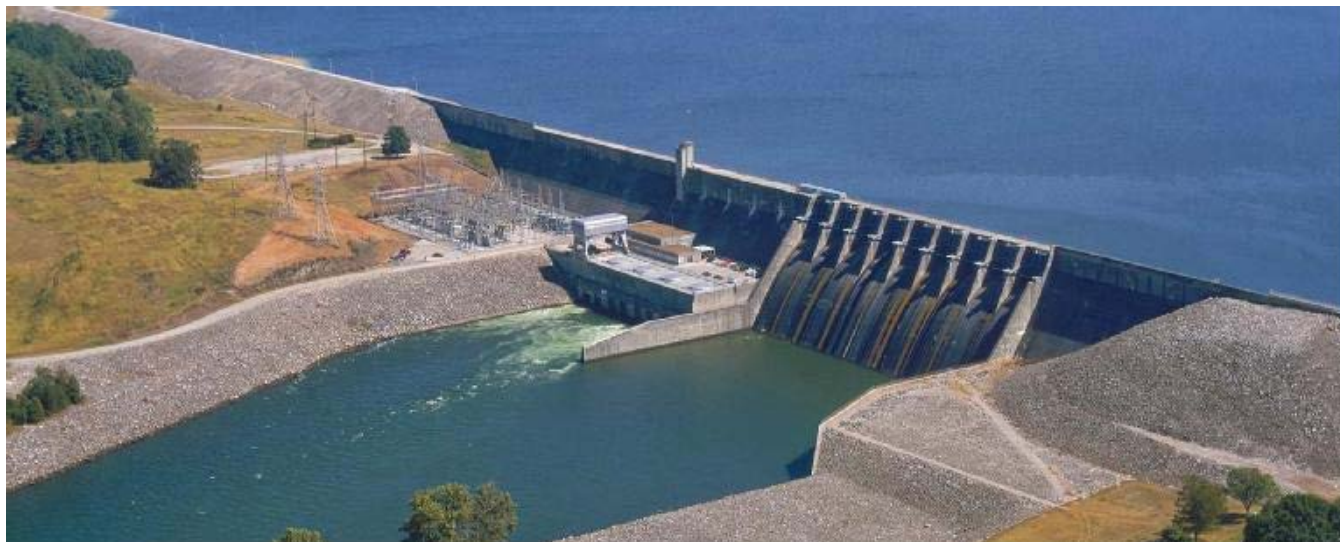
Figure 17-2 — Dam and Spillway of Hydroelectric Power Plant
