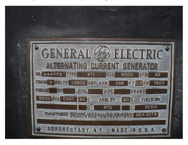
The Keokuk Energy Center contains 15 separate generators, each of which has a different nameplate attached. Each generator at Keokuk has a nameplate rating of less than 10 megawatts.
