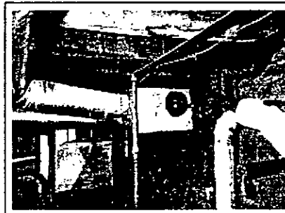
A wooden return system on a gravity furnace is not only leaky but also immediately adjacent to sundry volatile organic compounds. When the furnace is fired, fumes from these compounds can be whisked from the basement into the living area.
