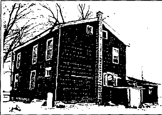
This farmhouse saved over 50 percent by air sealing, wall insulation, and furnace replacement.
