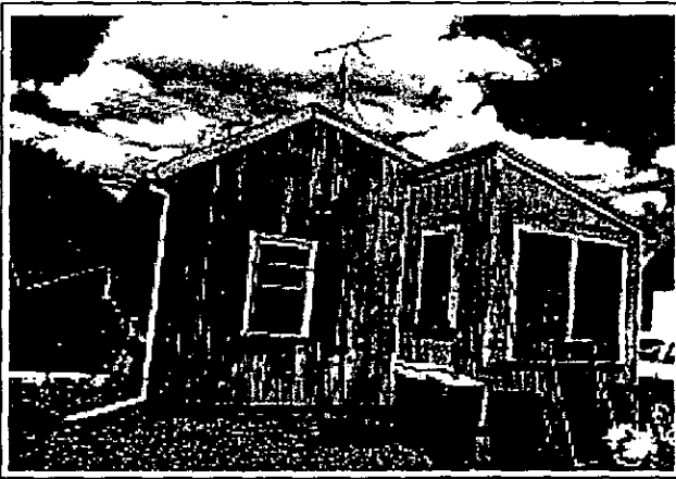
Joining the new to the old often causes trouble.
