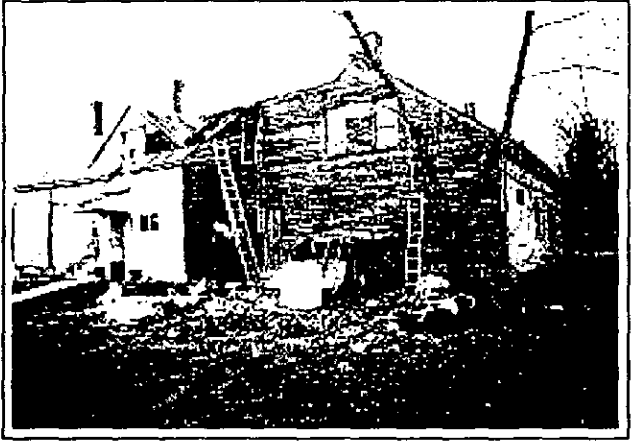
Movement of deteriorated foundation walls has opened large paths for air leakage.
