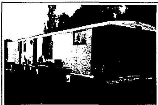
Mobile homes with poor foundations often develop major structural problems.
