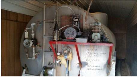
Missouri Utilities Water Tank (Exterior)
