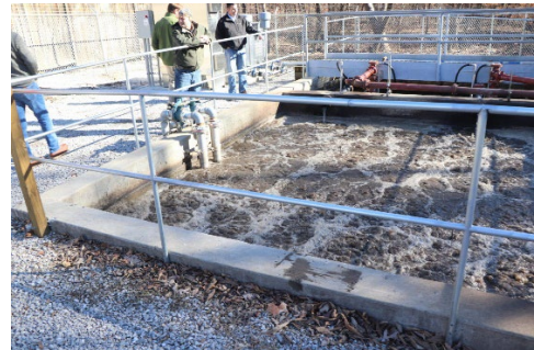
State Park Village – Aeration and Railing
