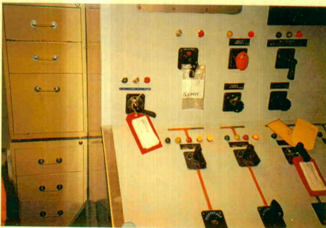
Photograph 12. Newly reinstalled DC oil pump control switch in control room (extreme left with red tag)
