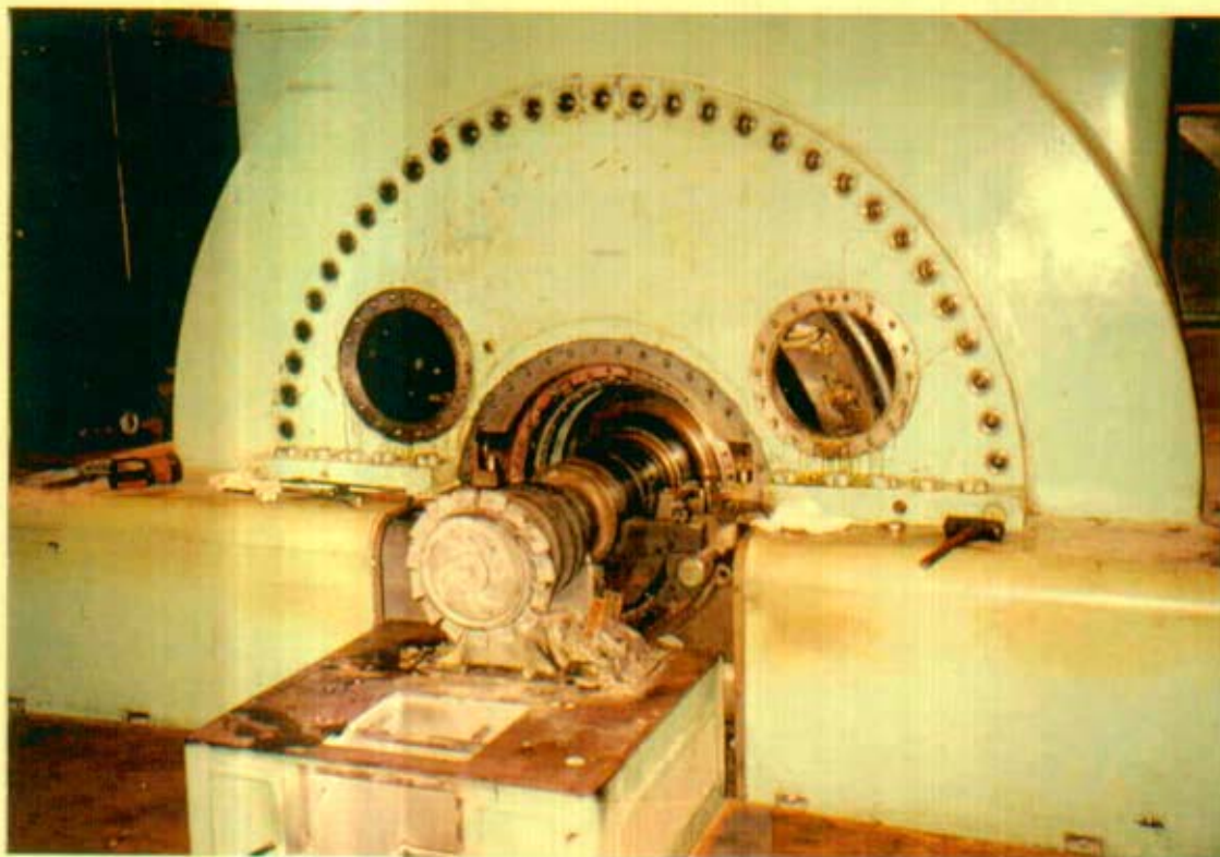
Photograph 4. No. 5 bearing on generator end
