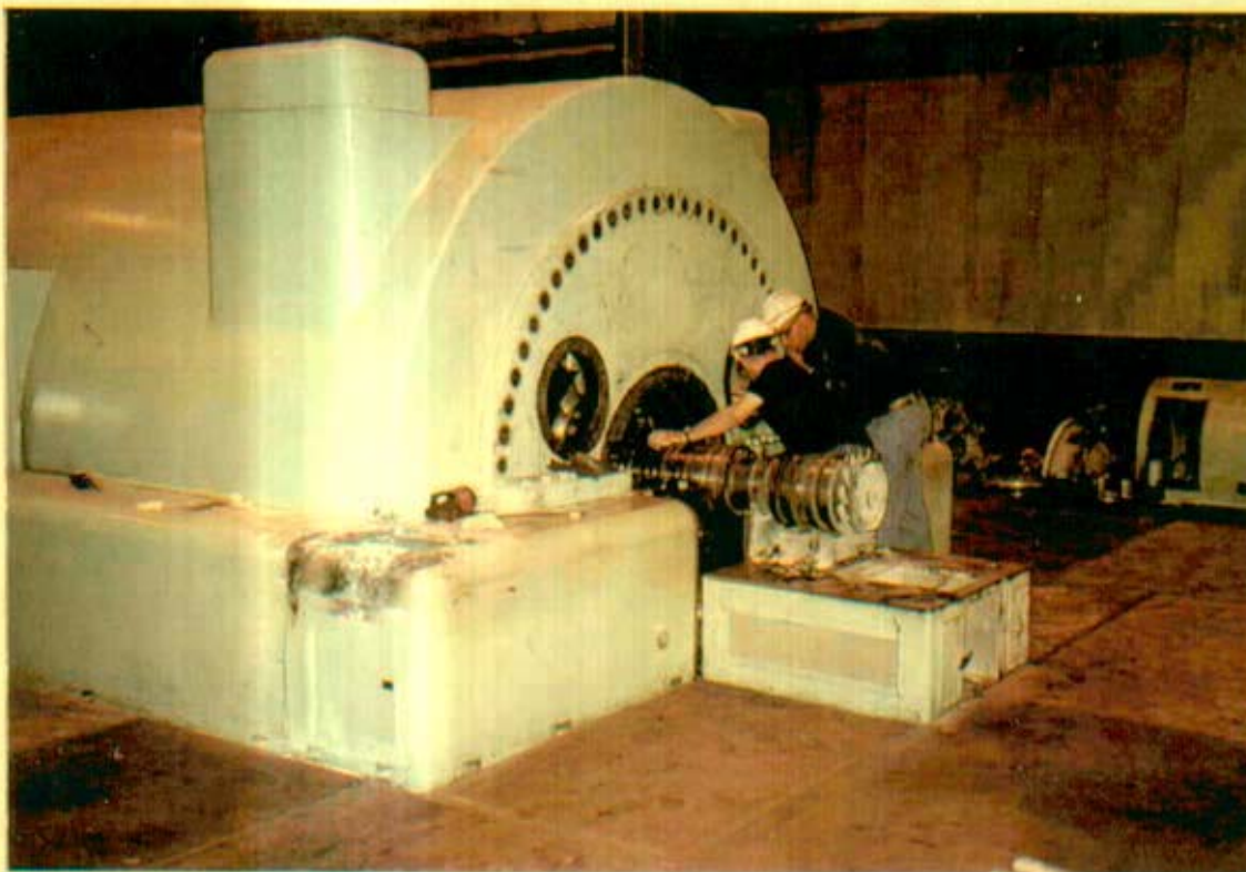
Photograph 1. Scorched paint on generator and No. 5 bearing damage
