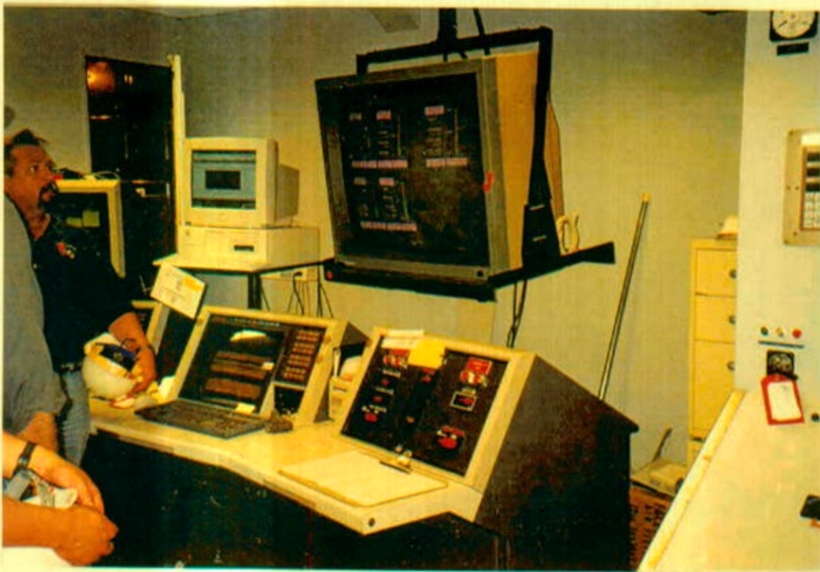
Photograph 13. Mark V operator interface and display in control room.
