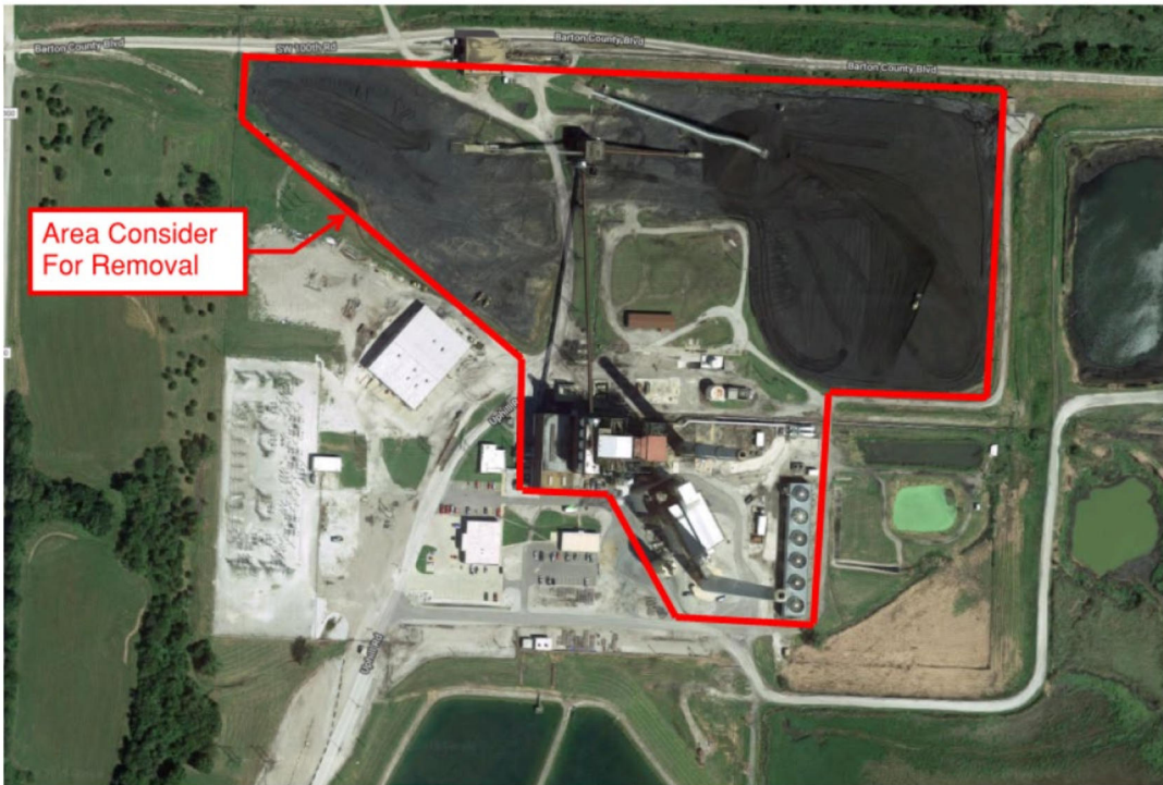
4 5 Figure 1 – Facilities Identified for Demolition
