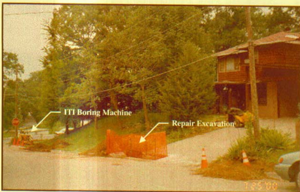
Photograph 1: 205 East Oak Street, incident site. Excavation in center of photograph was made to expose and repair the natural gas service line to 205 East Oak Street.
