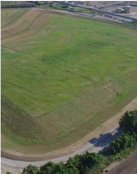
This ash basin at the Meramec Energy Center closed in the spring of 2018.
