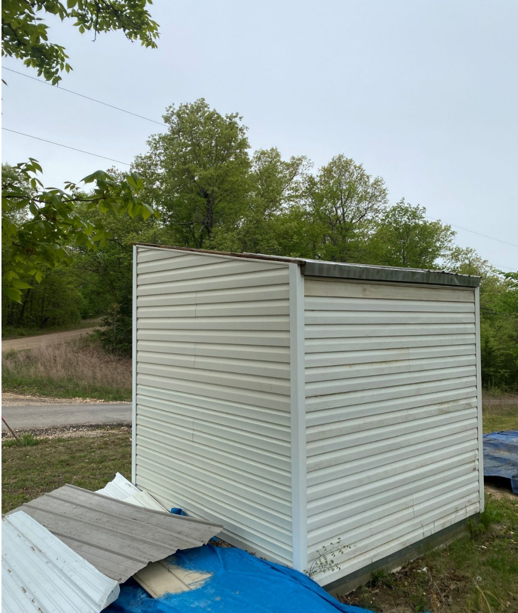
Figure 1 The Blevins Taylor Well has been out of service for over a year. According to an area service provider that I spoke with, it will not take much to repair it, but Blevins has not been able to do so. In the picture above you can see that it rests in disrepair with the well house missing its roof.
