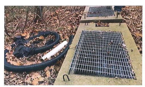
Construction and repair materials were left behind that should be removed from the site. The wire grate is not properly fitted. Note the leaves and rocks that are getting into the contact chamber and contaminating effluent, which should be
