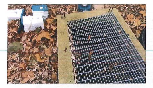
Empty chemical supply containers left behind that should be hauled to trash disposal. The edges of the bed are caked with leaf debris and a bush is growing out of the center of the far bed pictured. Also, note the leaves and rocks that are getting into the contact chamber contaminating effluent, which should be maintained and better protected for maintenance purposes. Leaves and construction repair material left on the bed can lead to premature failure of sand media.
