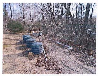
Trees are falling over the exterior fencing. All trees should be removed to maintain security of the wastewater facility.
