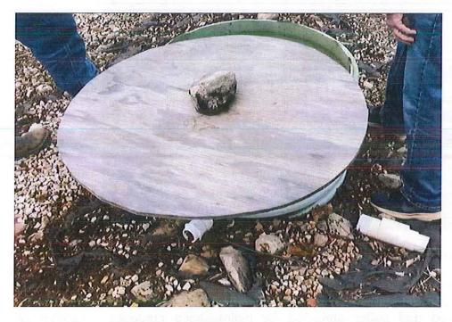
Unorthodox lid with rock holding it in place. This makeshift lid should be replaced with a proper lid. Also, construction and repair materials were left onsite that should be removed.
