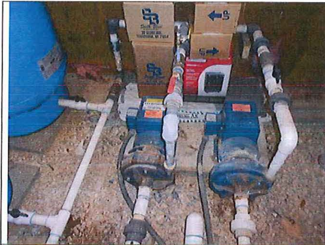
PHOTOGRAPH# 4 TAKEN BY: Darrell Barber ENTITY: Makalu Estates PERMIT: MO3031208 LOCATION: Inside well house DESCRIPTION: Two 5-hp booster pumps and related piping. DATE TAKEN: December 1, 2017 PROGRAM: Public Drinking Water Branch
