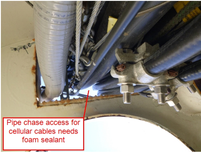
Coax cables mounted to ladder in dry tube
