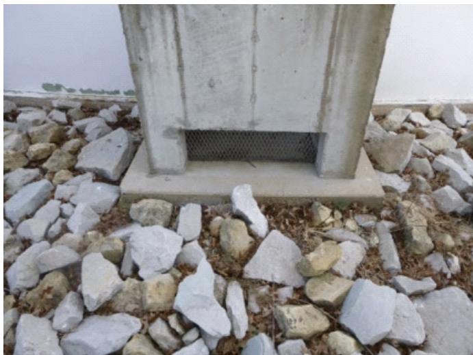
Overflow flap gate visible in concrete vault
