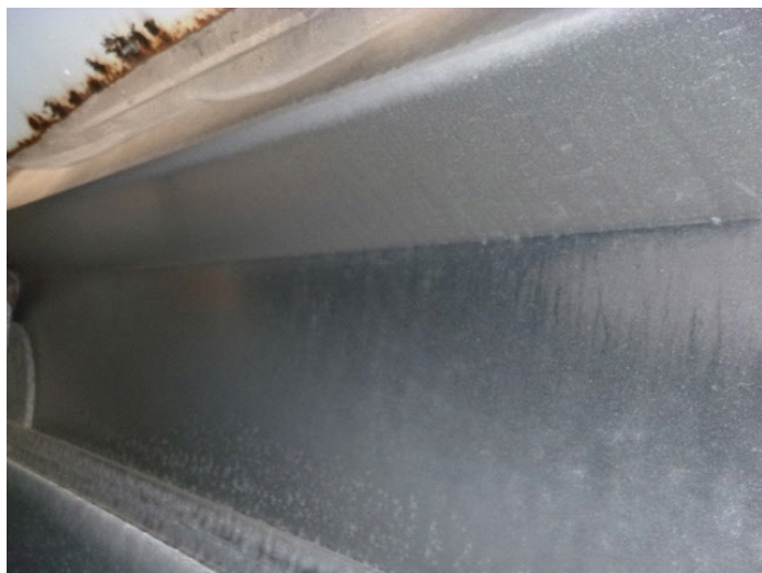
Surface rusting on overflow pipe
