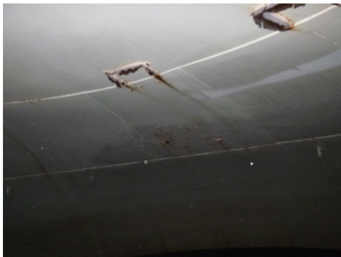
Rusting along overlapping roof plates
