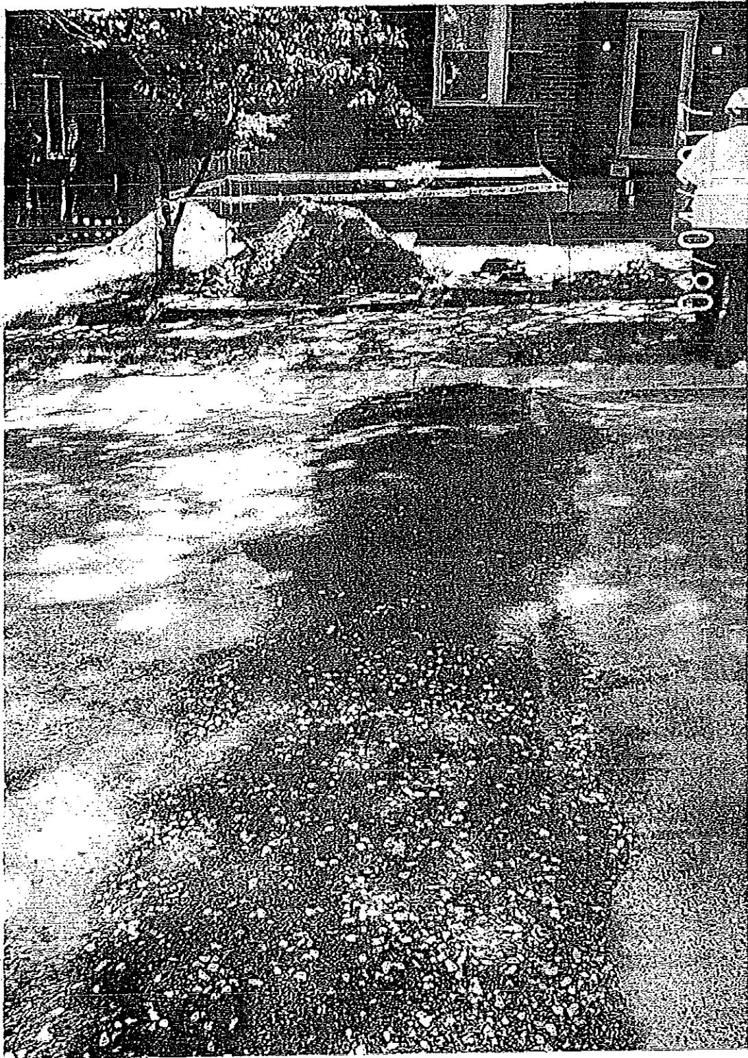
An example of a LSL replacement where the water main is on the opposite side of the street from the customer's home. This photograph is in the St. Louis County service area where the customer owns the entire service line.
