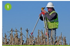
1 Surveys, soil borings, vegetation management and access roads
