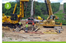
3 Dig structure holes
