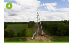
4 Lift structure into hole and backfill with concrete
