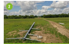
2 Assemble structure on the ground
